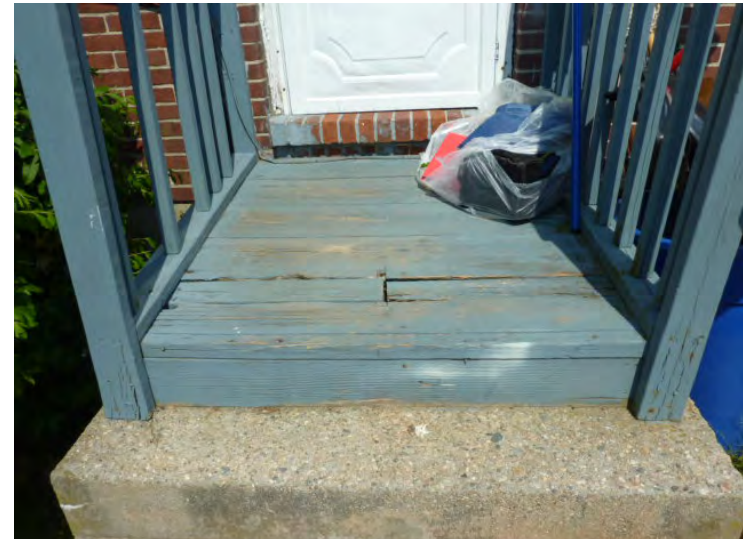
Deteriorated rear wood stairs and porches are shown to be replaced in Year 1.
