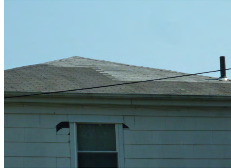
28 year old shingles are beginning to fail and are shown to be replaced early in the plan based on EUL and condition.
