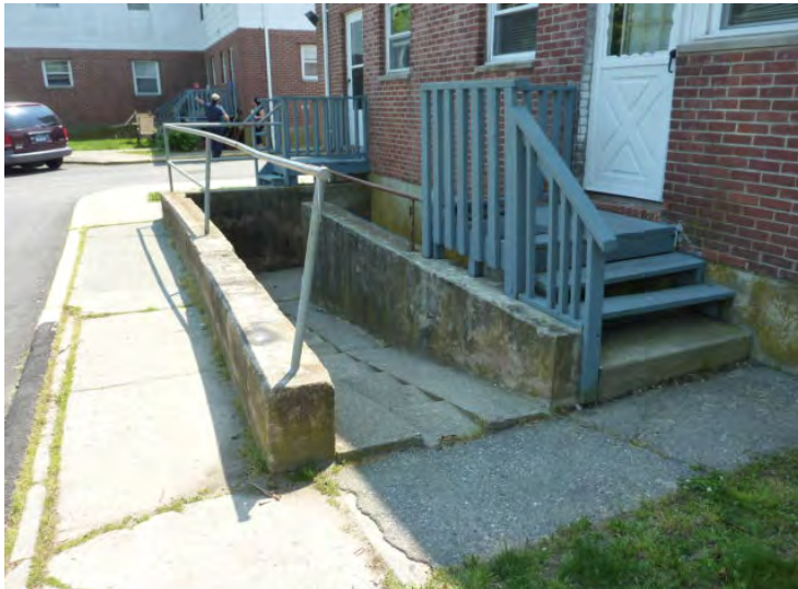
Repairs to concrete retaining walls and handrail at equipment ramp to basement at each building are shown mid-plan. Adjacent failing concrete is shown in Year 1.
