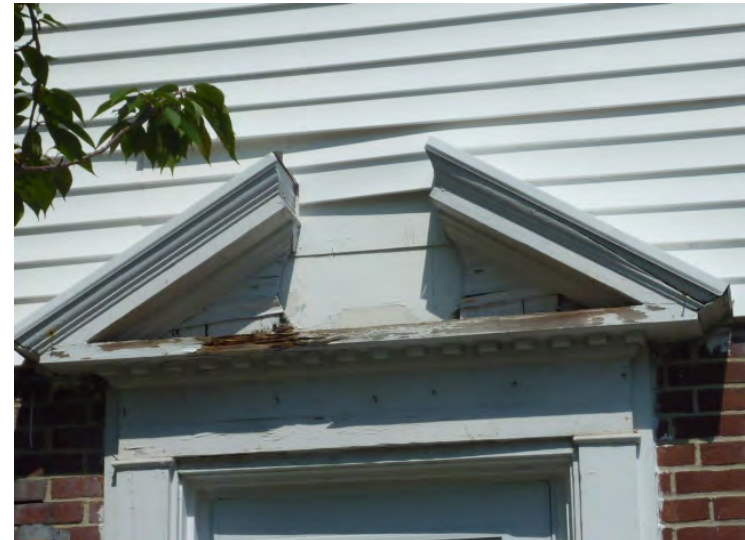
Typical deteriorating wood trim around all doors is shown to be replaced in Year1. Vinyl siding installed over possible asbestos cement siding at select location.
