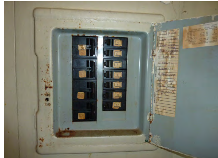
Electric panels are 40 years old and shown for replacement in Year 1.
