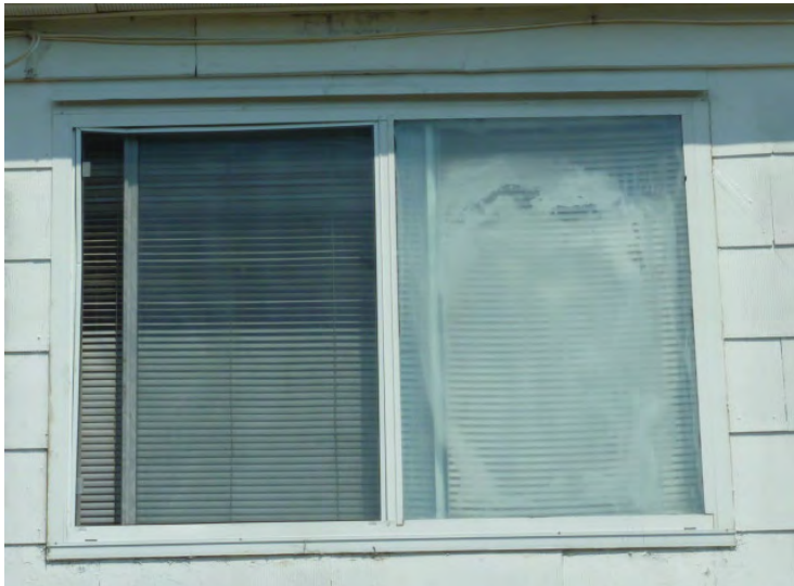
Typical failed seals at windows shown to be replaced in Year 1. Surrounding possible asbestos cement siding at second floor is also shown to be replaced in Year 1.
