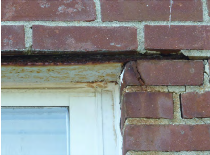
Typical flashing failure, rusting lintel and damaged brick is shown to be repaired in Year 1.
