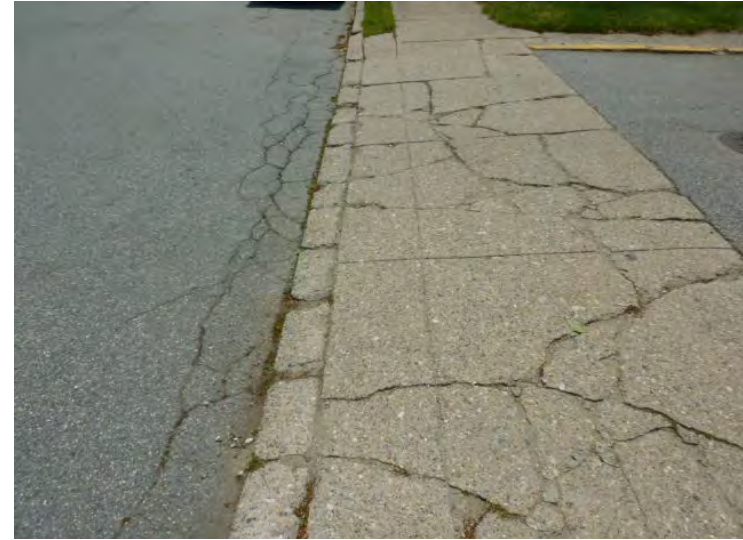
Typical cracking of asphalt paving on Third Avenue, and concrete curb and walk failure.
