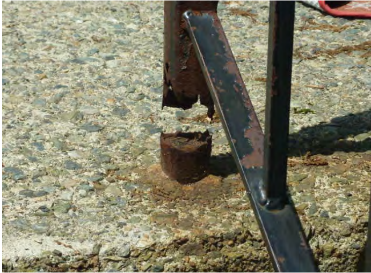
Handrails at all concrete stoops are shown to be replaced in Year 1.
