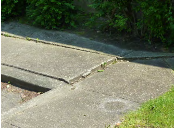
Typical of numerous trip hazards at concrete paving site-wide. All are shown to be eliminated in Year 1.
