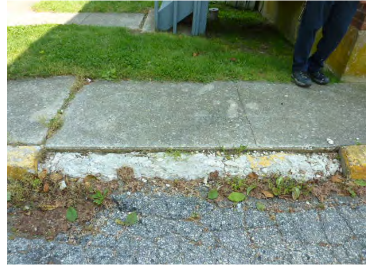
Typical deteriorated concrete curb, worn concrete walk, and trip hazards site-wide. All are shown to be eliminated in Year 1.
