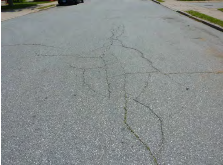
Typical cracking of asphalt paving on Third Avenue. The asphalt street paving and the adjacent concrete curbs and walks are the responsibility of the owner.
