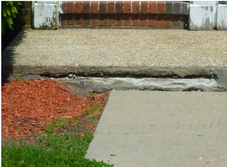
Concrete stoops are failing at rusting reinforcing bars and have been repeatedly patched. Replacement is shown in Year 1.
